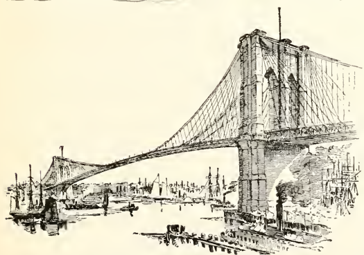
EAST RIVER BRIDGE
